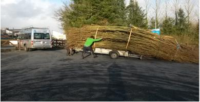
The task of build the structure began in February 2016. Stage one was building the pillars that would form the A frames of the structure. This was done by banding together lengths of Willow in one direction and inverting the same amount in the opposite direction to create stability.
